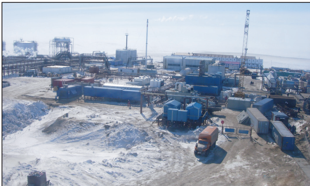
The Tedinskoe oil field is operated by Lukoil Sever and the OP16s use wellhead gas to supply 1.8 MWe each.
